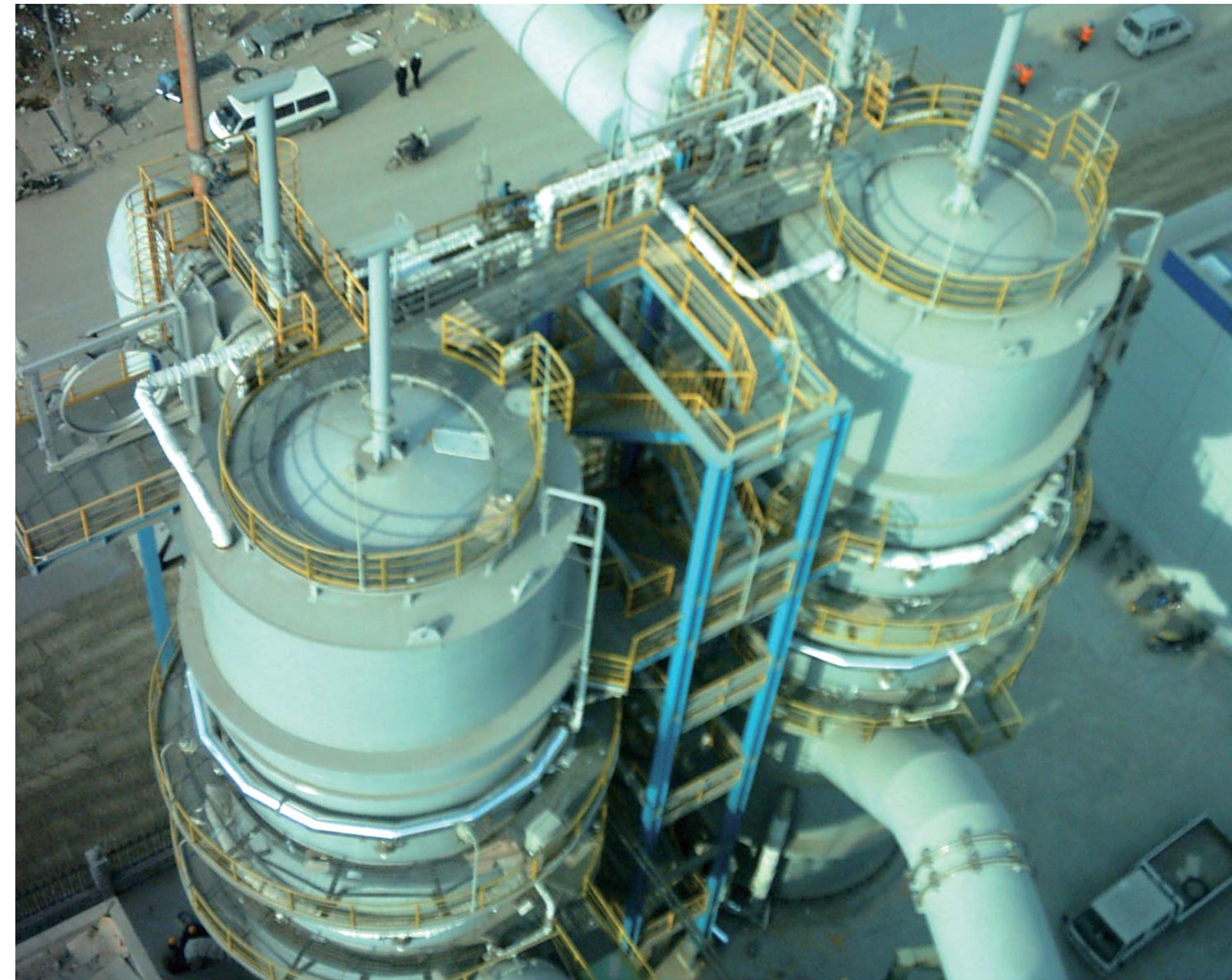
转炉煤气干法除尘煤气冷却器 Dry dedusting cooler for converter gas
