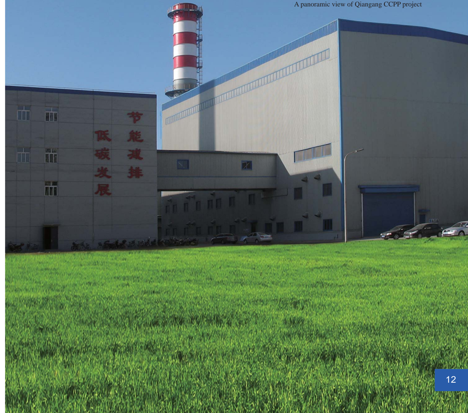
迁钢CCPP工程全景 A panoramic view of Qiangang CCPP project
