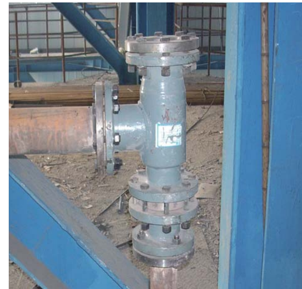
可调补气器，精确控制输送气量 Adjustable air make up device, for accurate control of the transport gas flow
