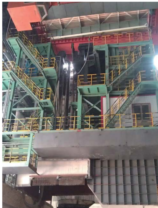
铁水脱磷 Hot metal dephosphorization
